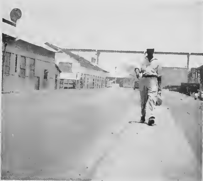
This man is walking where tube bundles will be repaired and tested when the addition to the old shop building is finished. This section (see 9 on drawing on page 4) will be 3,500 sq. ft. of storage space. Pipe and welding shops at left were dismantled.
